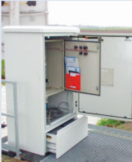
Level measurement in a sewer and sequential control of a sluice Protection is provided by the robust CS modular enclosure.
